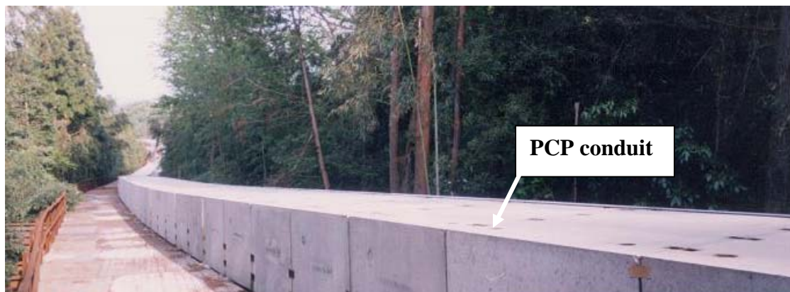
(b) PCP conduit outside the Tunnel
